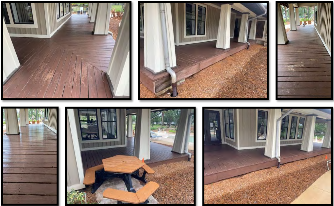
The deck in front of the gym was stained.
