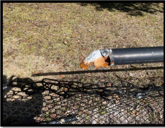
Cut off rusted portions of the top rail out at the multi-purpose fields
