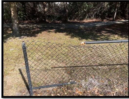
Cut off rusted portions of the top rail out at the multi-purpose fields
