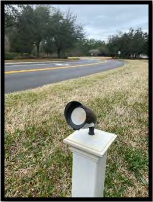
New light installed at marquee
