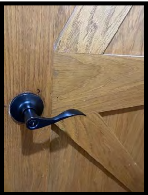
New interior door handles are installed in the bathrooms.
