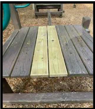
Several planks at playground replaced
