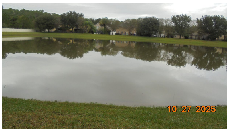
Pond 13: Pond was in good condition. Water level is normal.
