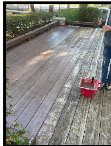
There were some drawings on the screens that were covered with new paint. We are applying a sealer on the deck and all the brown colored wood.
