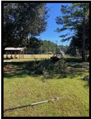
Trimming limbs that might cause interference with our systems.
