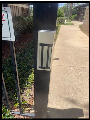
Replaced old mag lock with new.
