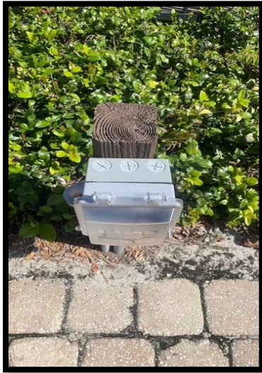
Replaced old damaged GFCI and enclosure with new.
