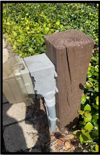
Replaced old damaged GFCI and enclosure with new.
