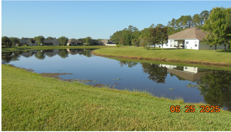
Pond 8: Pond was in good condition. The water level is normal. Fountain running normally.
