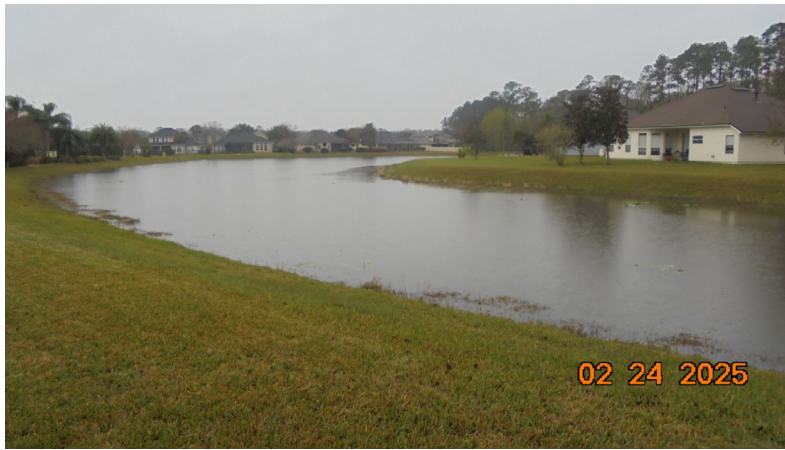
Pond 8: Pond was in good condition. The water level is normal. Fountain running normally.
