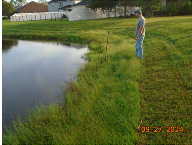
Cleaned fish barrier on outflow structure.
