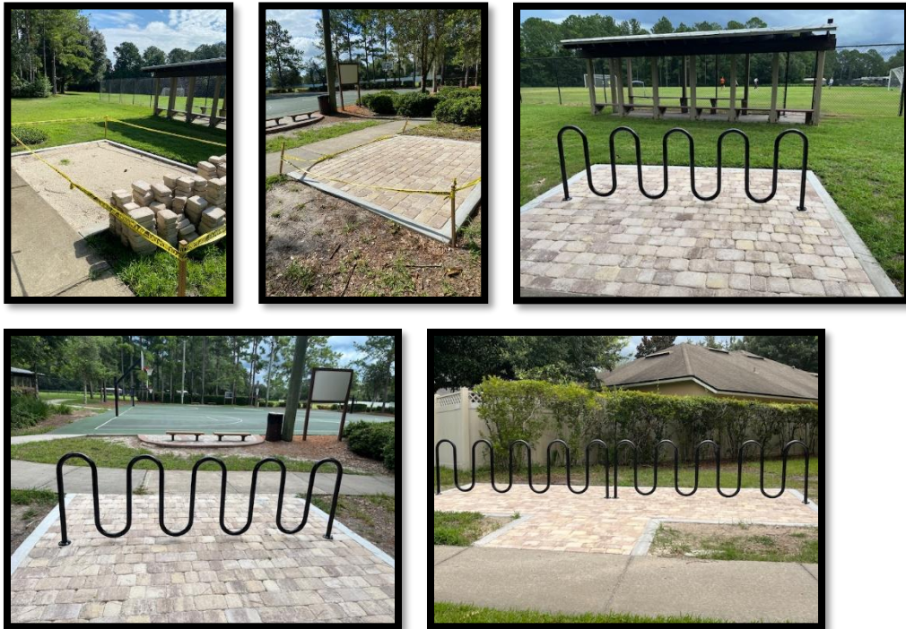
The bike racks have been installed.
