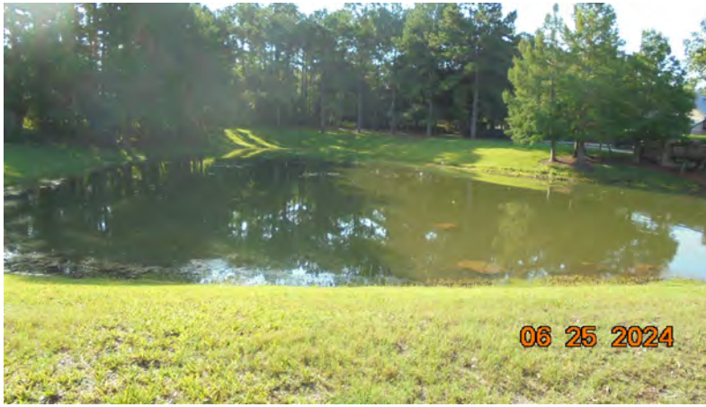
Pond 5: Pond was in good condition. The water level is normal.
