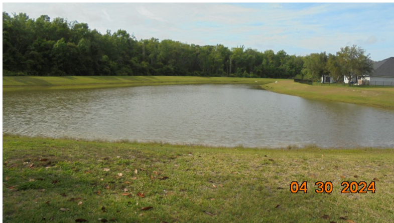
Pond 9: Pond was in good condition. The water level is good.
