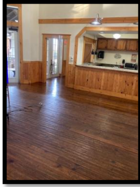
Stained the Heritage Room floor to blend scratches.
