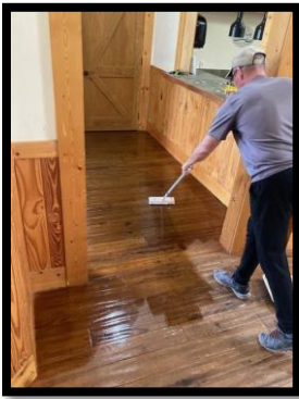
Stained the Heritage Room floor to blend scratches.
