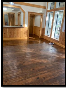
Stained the Heritage Room floor to blend scratches.
