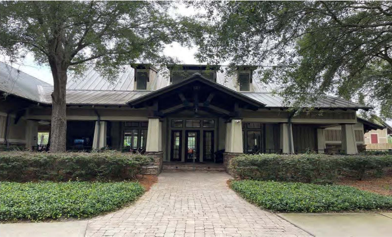
Amenity Center – Entrance (06-26-23)
