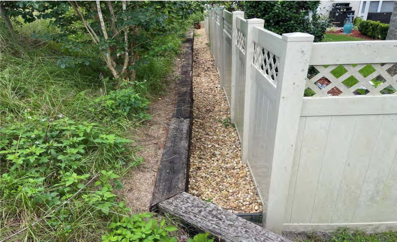
CDD Owned Retaining Wall at River City Street Cul-de-Sac (06-26-2023)
