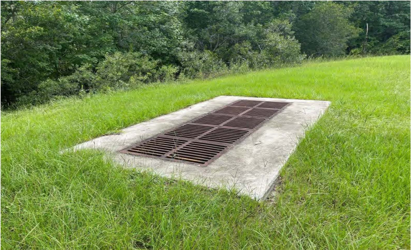
Storm Water Management Facility No. 5 Control Structure (06-26-23)
