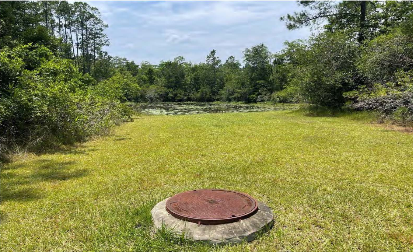
Dispersion Basin Storm Water Management Facility No. 1 (06-26-23)
