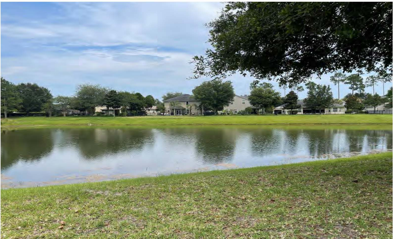
Storm Water Management Facility No. 6 (06-26-23)
