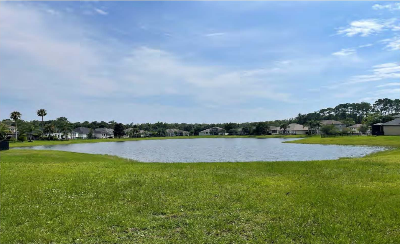
Storm Water Management Facility No. 8 (06-26-23)
