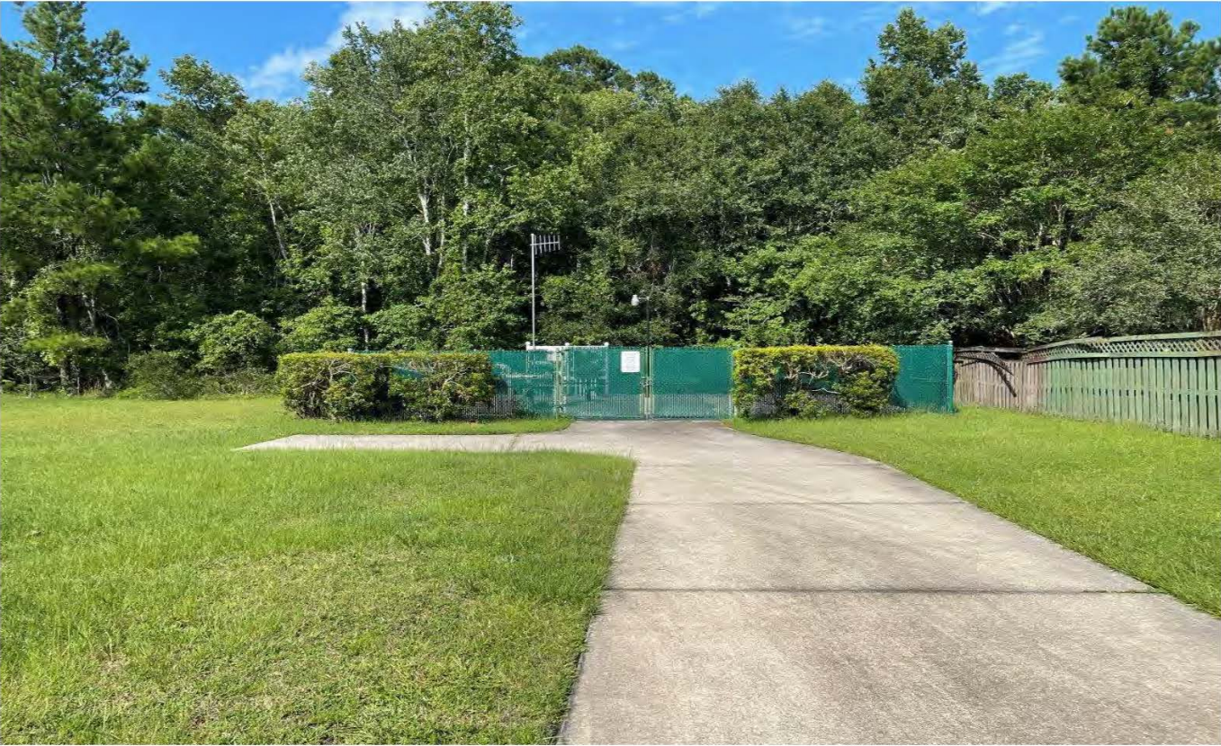
Lift Station on Silver Glen Avenue (06-26-23)
