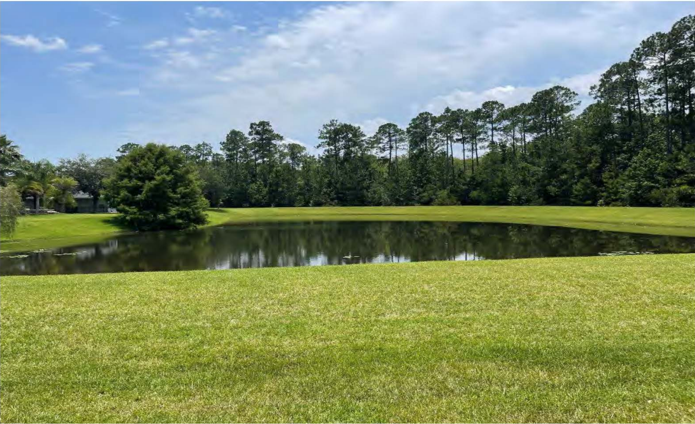
Storm Water Mangement Facility No. 1 (06-26-23)
