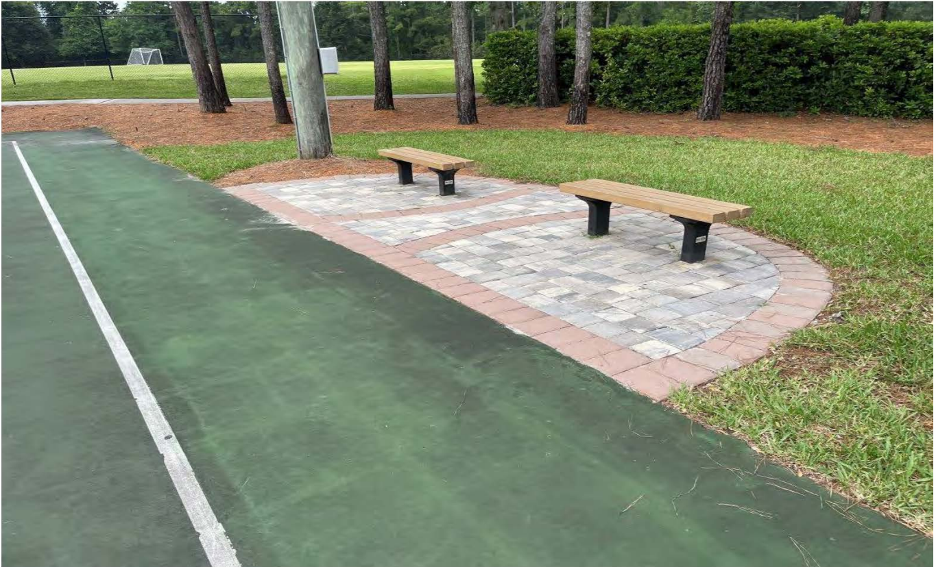
Amenity Center – Pavers recently installed for Basketball Benches (06-26-23)
