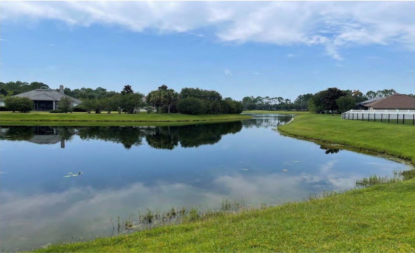
Storm Water Management Facility No. 5 (06-26-23)
