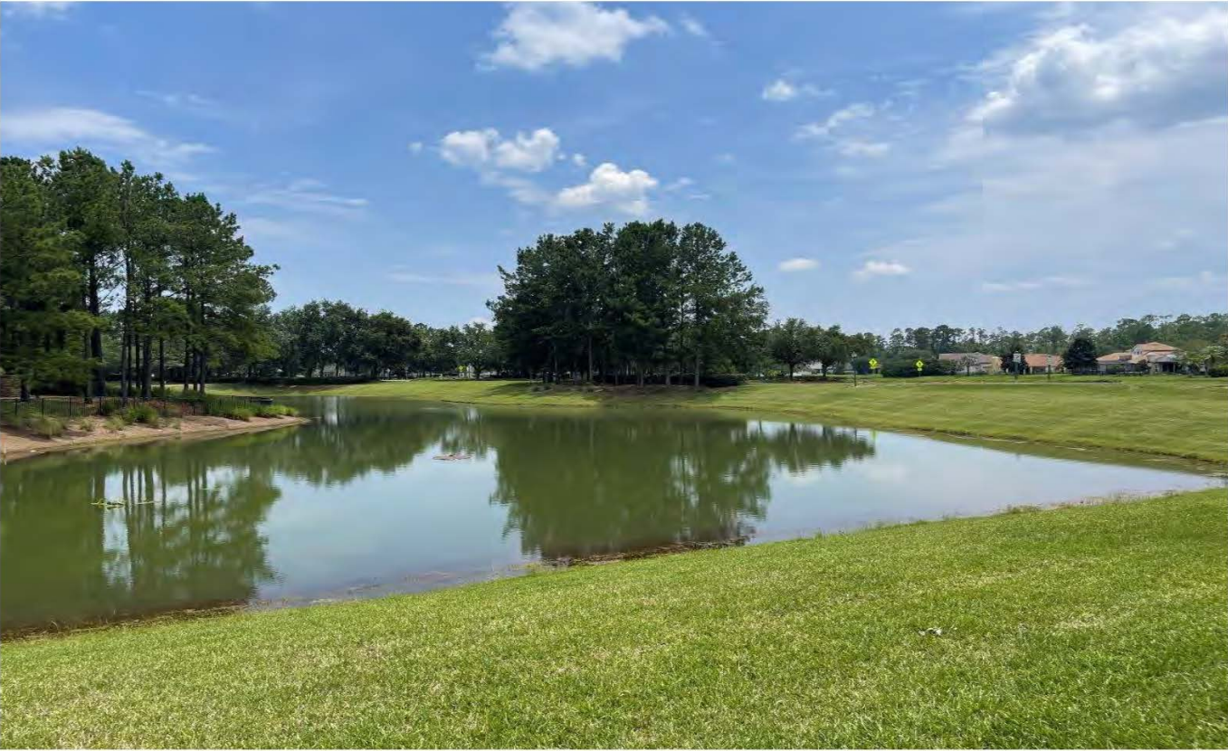
Storm Water Management Facility No. 4 (06-26-23)
