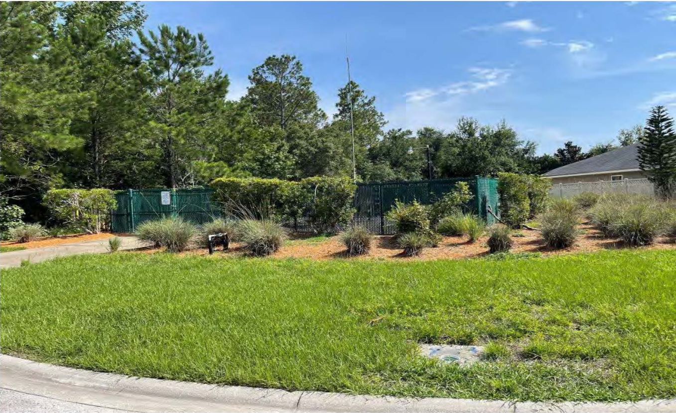
Lift Station on Cowford Ferry Court (06-26-23)
