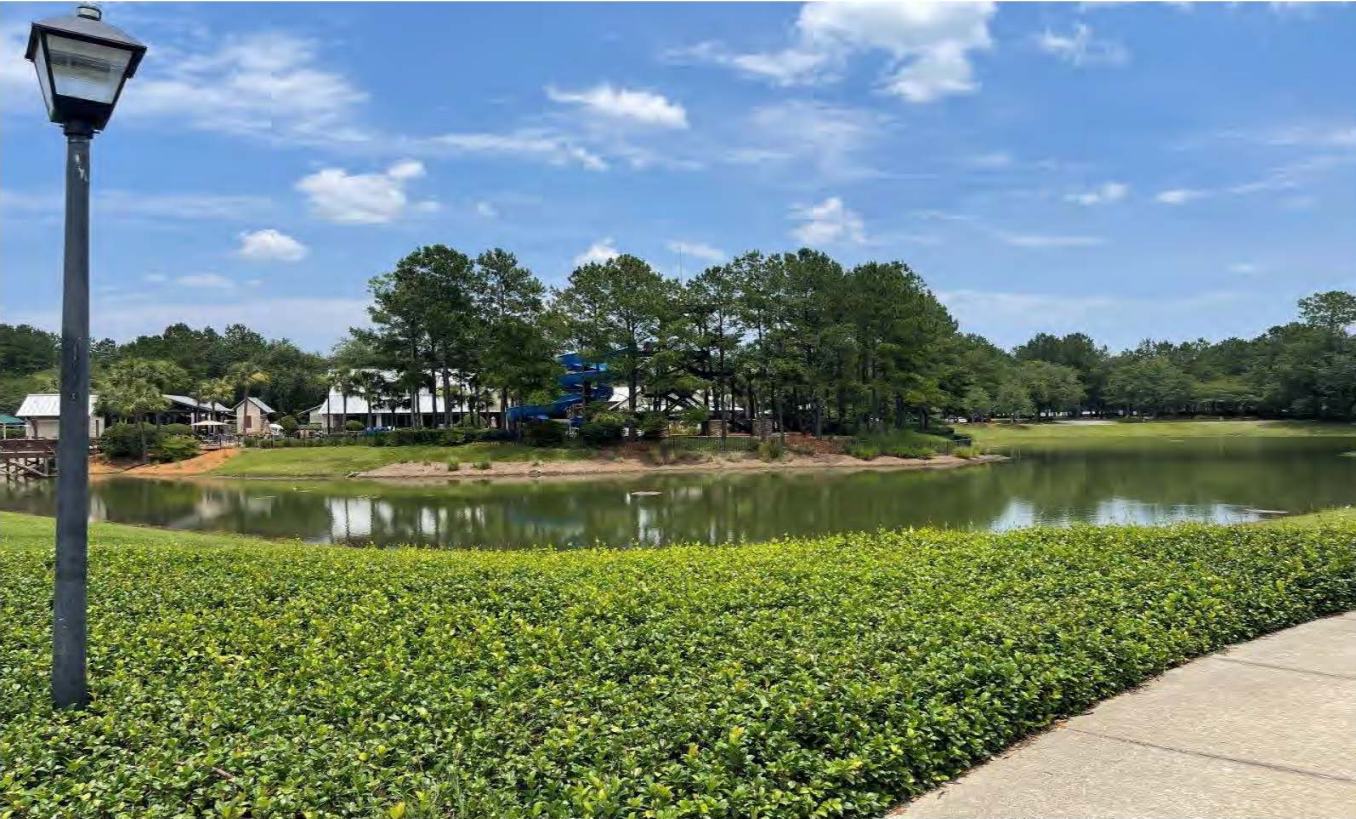
Storm Water Management Facility No. 4 adjacent to the Amenity Center (06-26-23)
