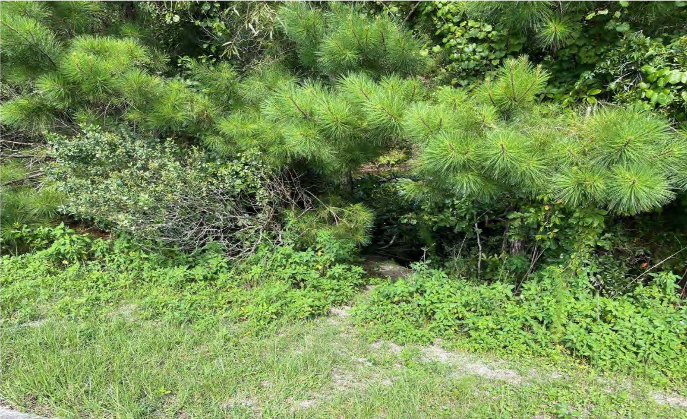
Storm Water Management Facility No. 10 – Dispersion Basin (06-26-23)
