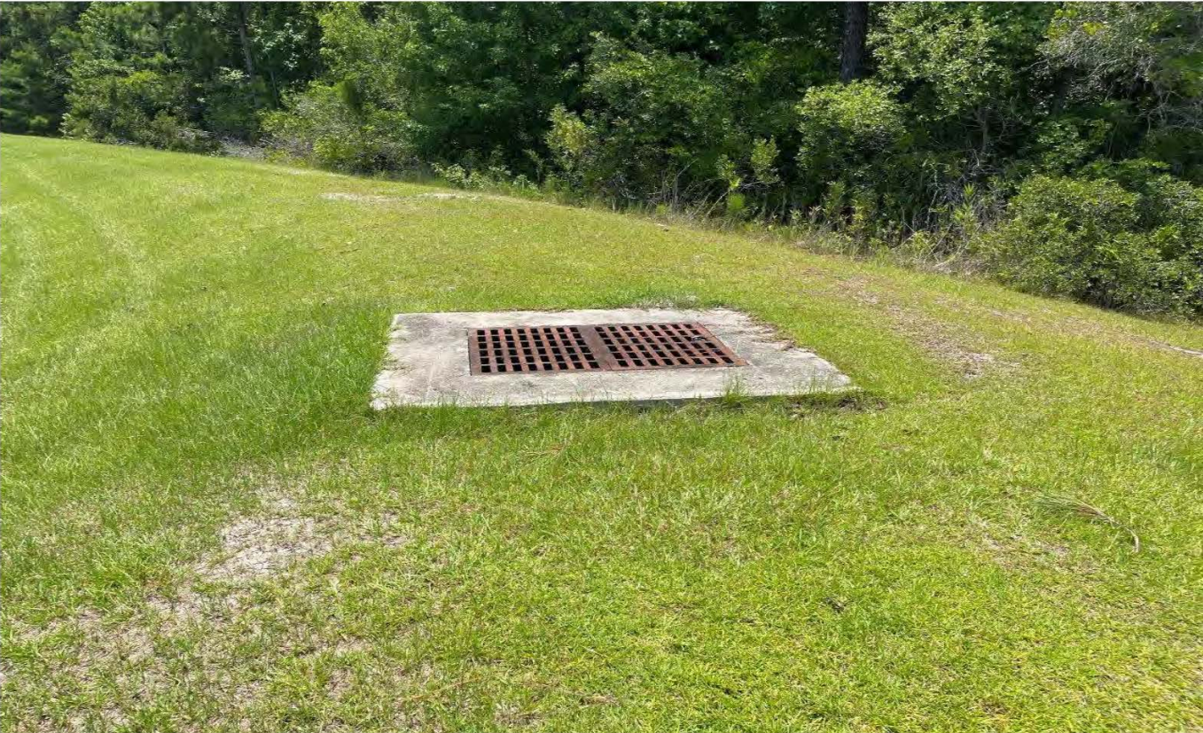
Storm Water Management Facility No. 1 Control Structure (06-26-23)
