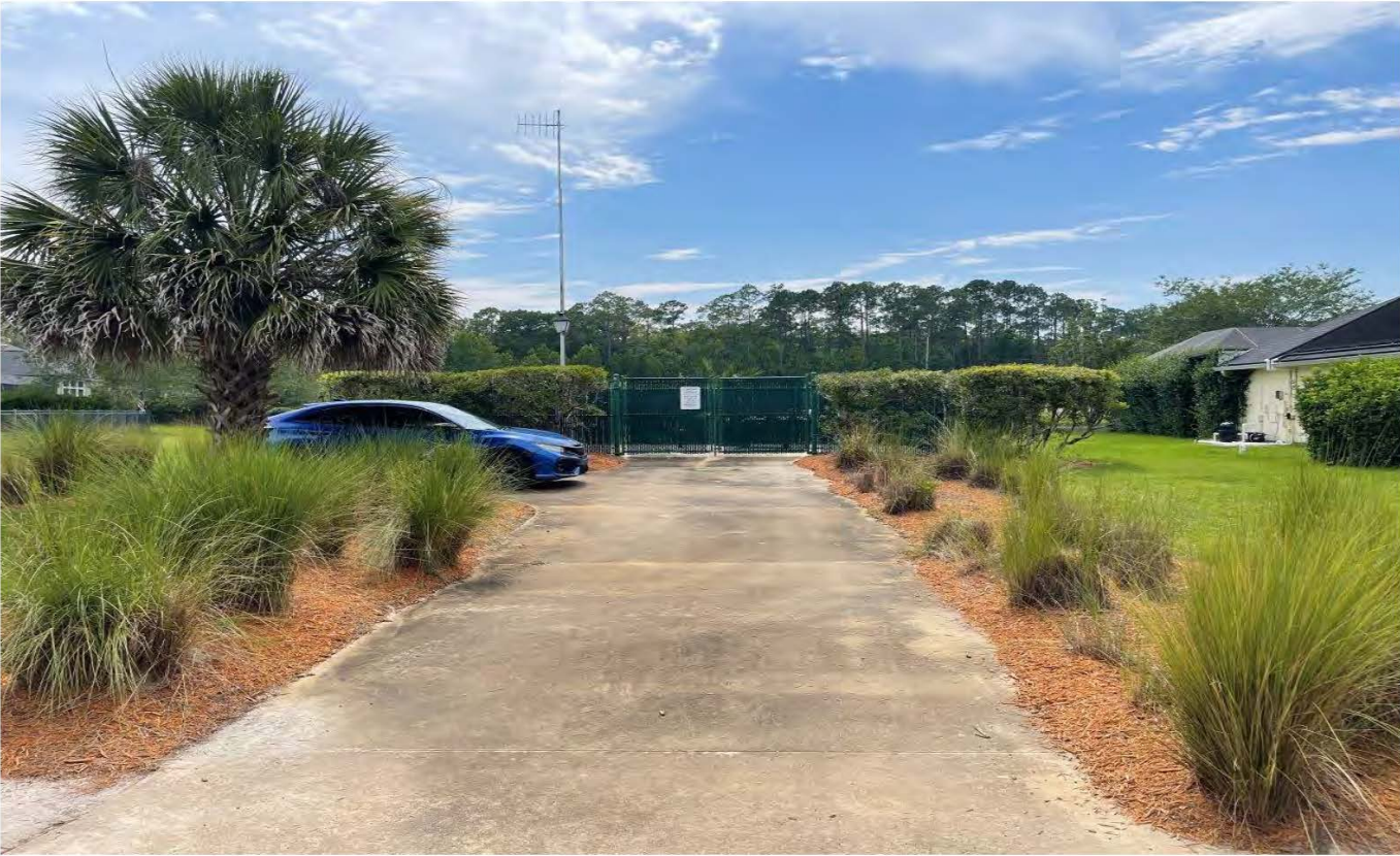
Lift Station on Swallowtail Lane (06-26-23)
