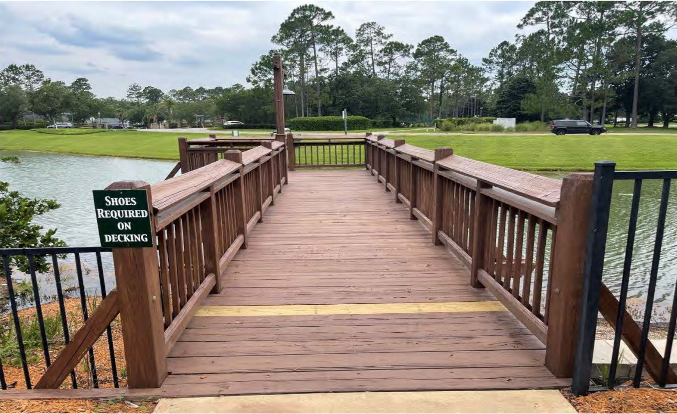
Amenity Center – Pedestrian Dock over Storm Water Management Facility No. 4 (06-26-23)
