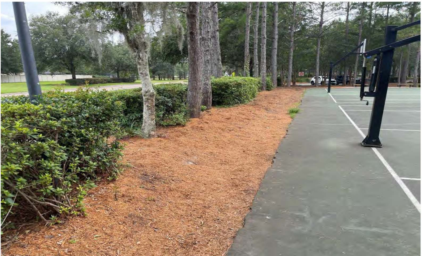
Amenity Center – Drainage Swale Adjacent to Basketball Court (06-26-23)
