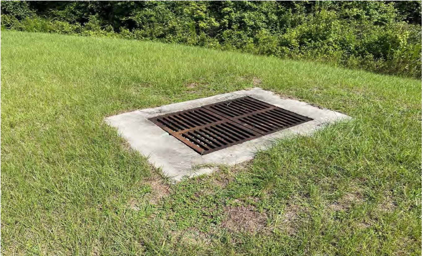
Storm Water Management Facility No. 9 – Control Structure (06-26-23)
