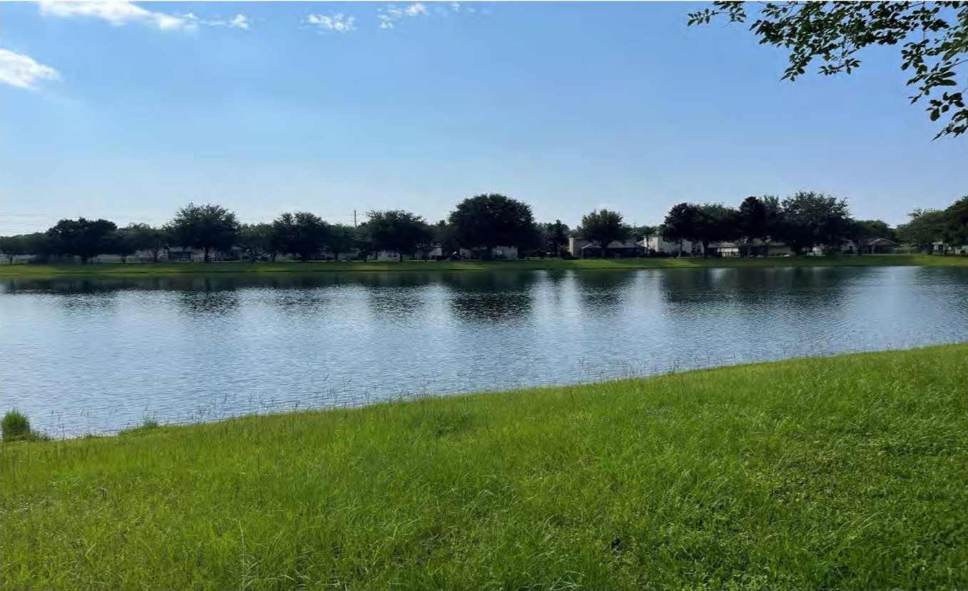
Storm Water Management Facility No. 12 (06-26-23)
