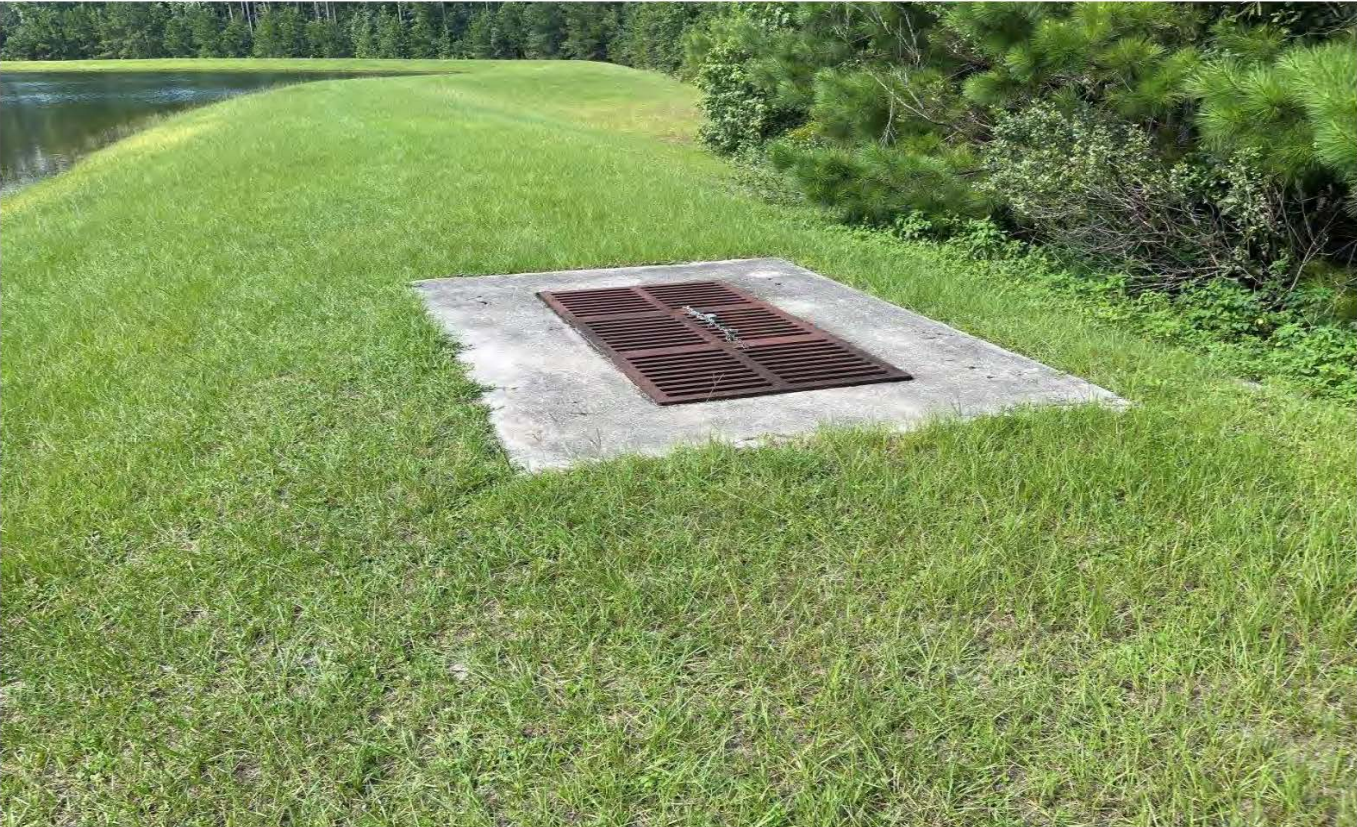
Storm Water Management Facility No. 10 – Control Structure (06-26-23)
