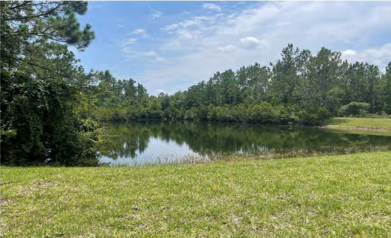
Storm Water Management Facility No. 3 (06-26-23)
