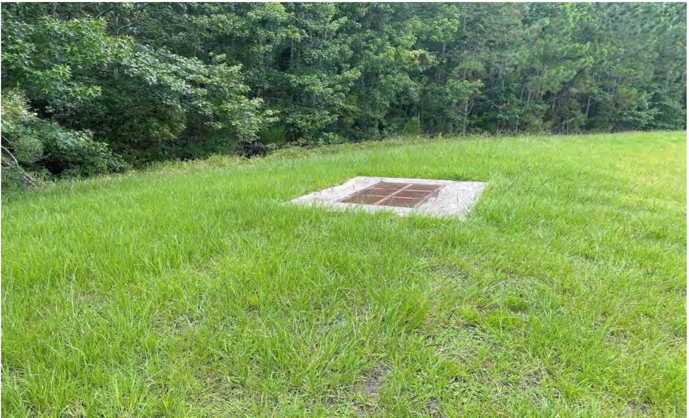
Storm Water Management Facility No. 7 – Control Structure (06-26-23)
