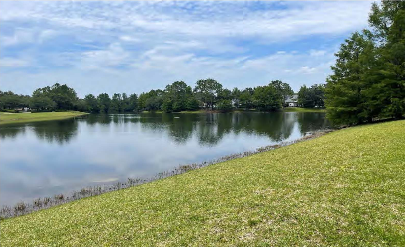
Storm Water Mangement Facility No. 2 (06-26-23)
