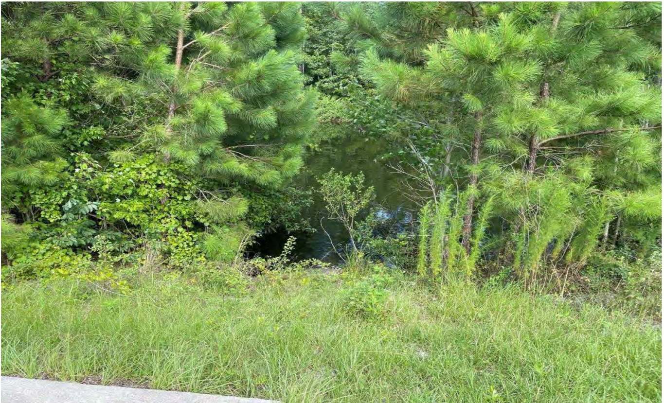
Storm Water Management Facility No. 11 – Dispersion Basin (06-26-23)
