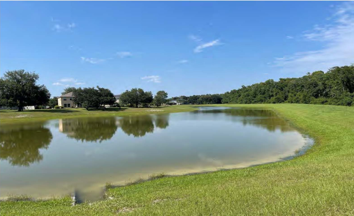
Storm Water Management Facility No. 9 (06-26-23)
