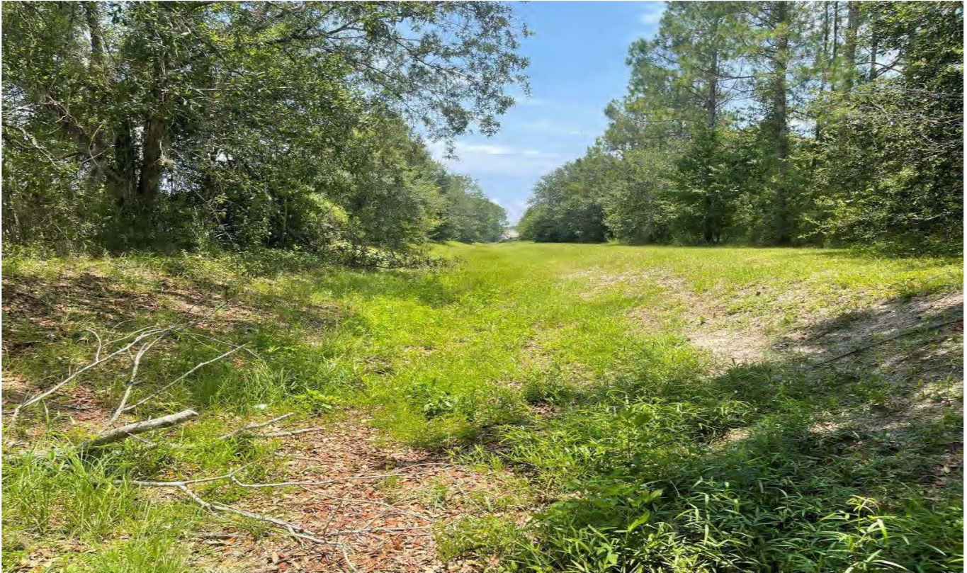
Drainage Swale (Northerly end of project near County Road 13) (06-26-23)
