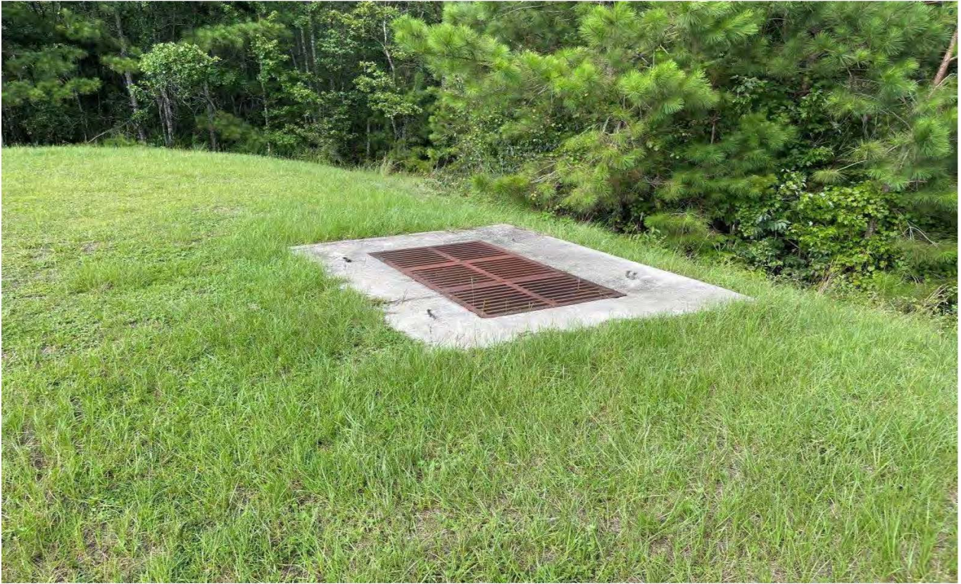
Storm Water Management Facility No. 11 – Control Structure (06-26-23)
