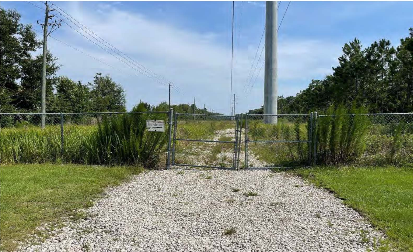
FPL Easement Access along Heritage Landing Parkway (Facing North) (06-26-23)
