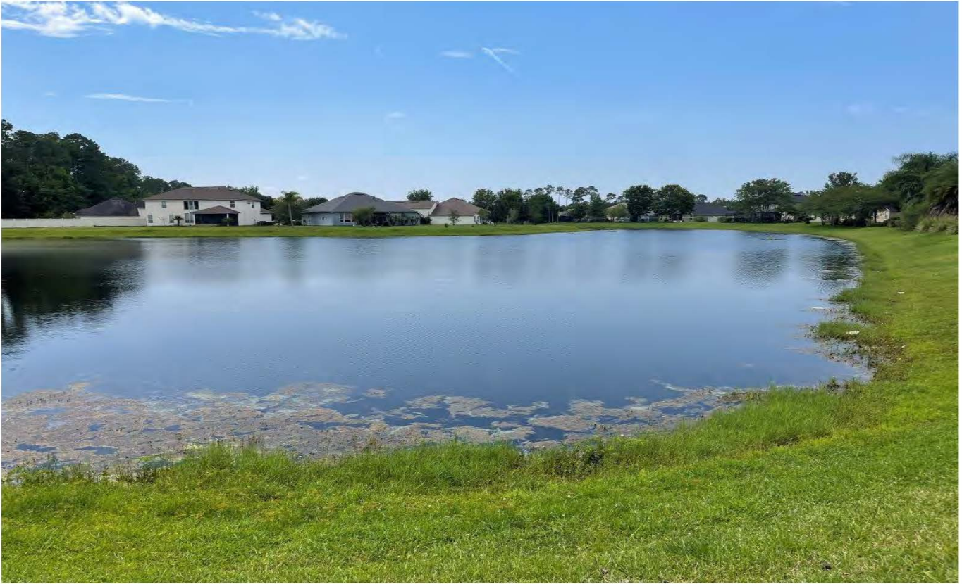
Storm Water Management Facility No. 7 (06-26-23)
