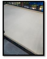
One of the items on the Adkins list that needed to be completed/redone was the waterproofing of the landings. The landings were sanded/grinded with a diamond wheel disc. The different layers of waterproofing were laid down.
