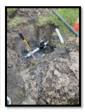
The line broke right at the old irritrol valve. The valve was replaced at the same time with a new one.
