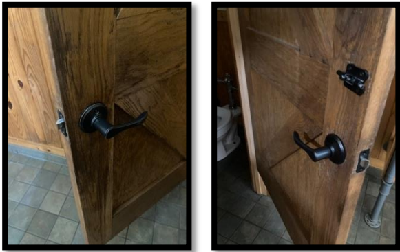
New door handle installed at men's bathroom
