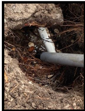
3 additional irrigation breaks were repaired by BrightView.
